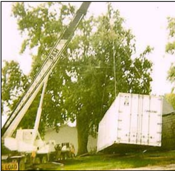
The crane lifts the shop from its old location.
